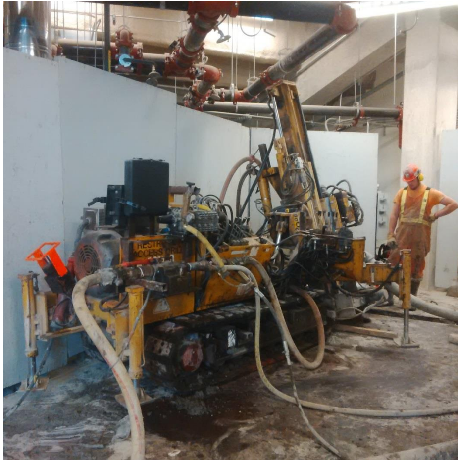
FIGURE 6: MICROPILE DRILLING IN AREA A
