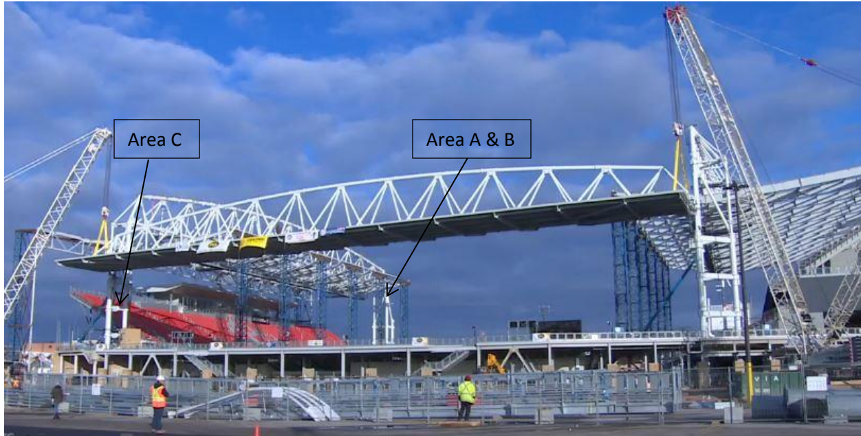
FIGURE 1: BMO FIELD RENOVATIONS IN PROGRESS, LOOKING NORTH
