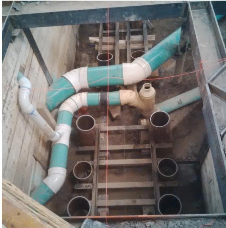
FIGURE 5: RELOCATED UNDERGROUND SERVICES & DRILLING TEMPLATE
